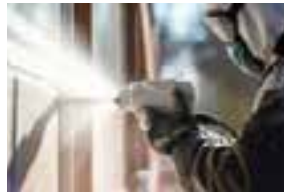
Sandblasting for paint stripping
